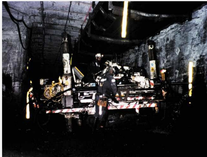
Figure 2 – Gas drainage drilling rig at Metropolitan Colliery
