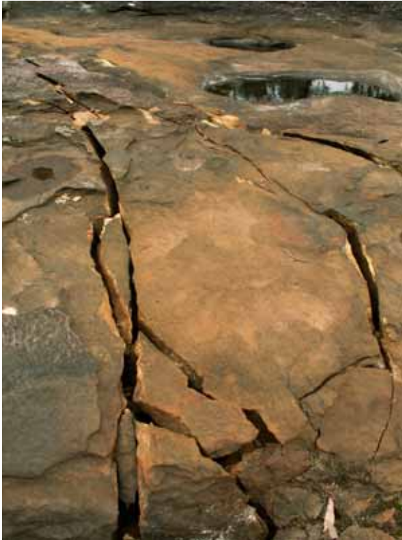
Waratah Rivulet - cracked by longwall mining
